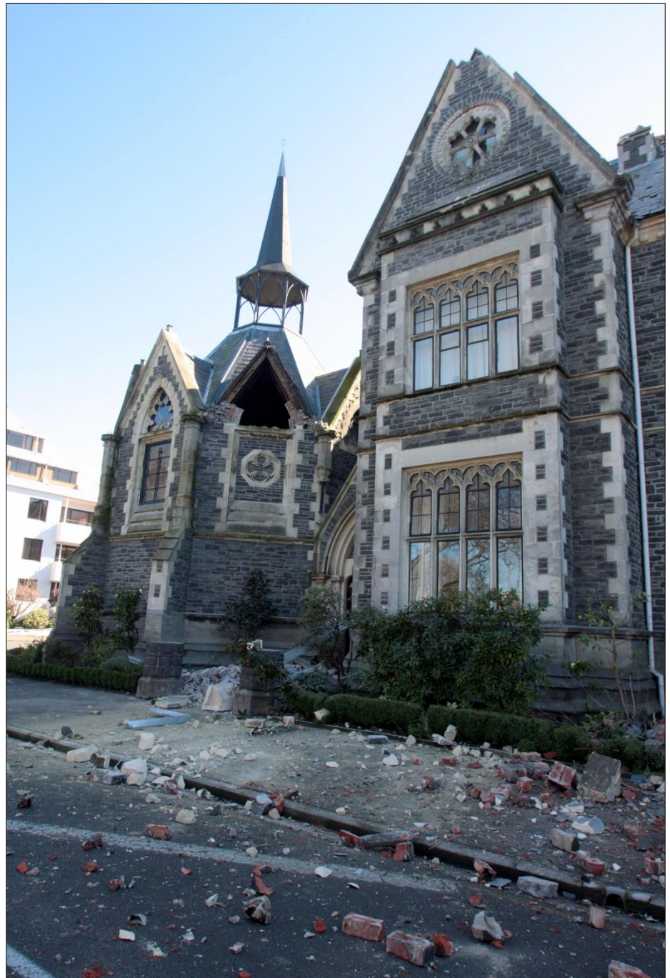
Damage to the octagonal room makes it the second time round for Cranmer Square's 1875 former Normal School, now Cranmer Court, which lost two towers after an earthquake in 1928.
