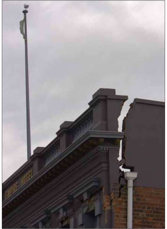
Clockwise from top: Damage to the gable end of the 1905 nave extension, Holy Trinity, Avonside (Category I); detached facade, Empire Hotel, Lyttelton; the only fire-damaged building in the CBD in Worcester St; and one of the lucky ones in Hereford St. Photos: Ann Devereaux
