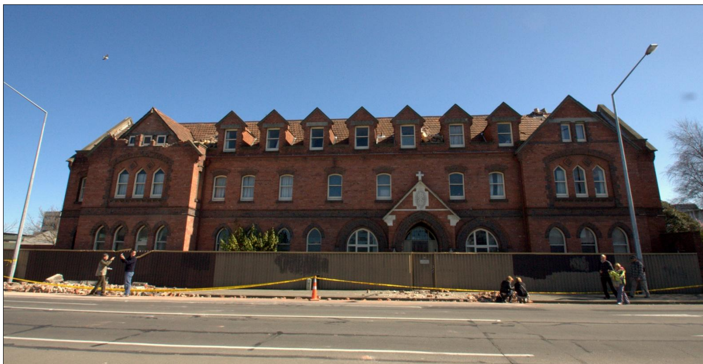
Below: Damaged. The Category 1 Community of the Sacred Name in Barbados Street, (J.G. Collins, 1911-12, with earlier sections by B.W. and C.J. Mountfort), has sustained damage front and rear. Photos: Ann Devereaux
