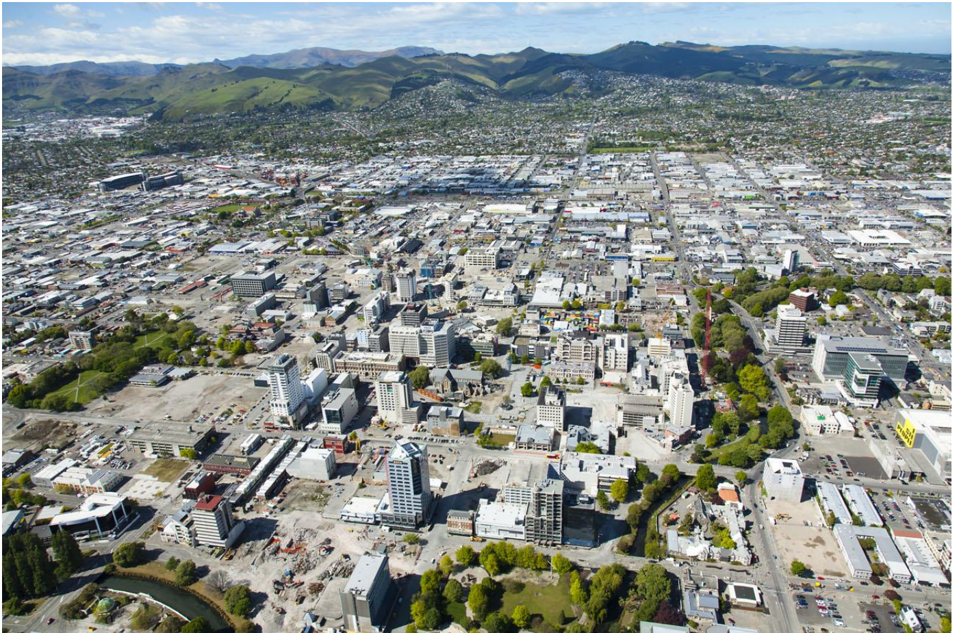
Looking south towards the Port Hills with Colombo Street centre picture, from above the Town Hall, the effect of 14 months of demolition can be appreciated. The two leaning high rises overlooking Victoria Square's flagstaff await demolition. The Canterbury Provincial Buildings, now secured are in the lower right of the picture.
