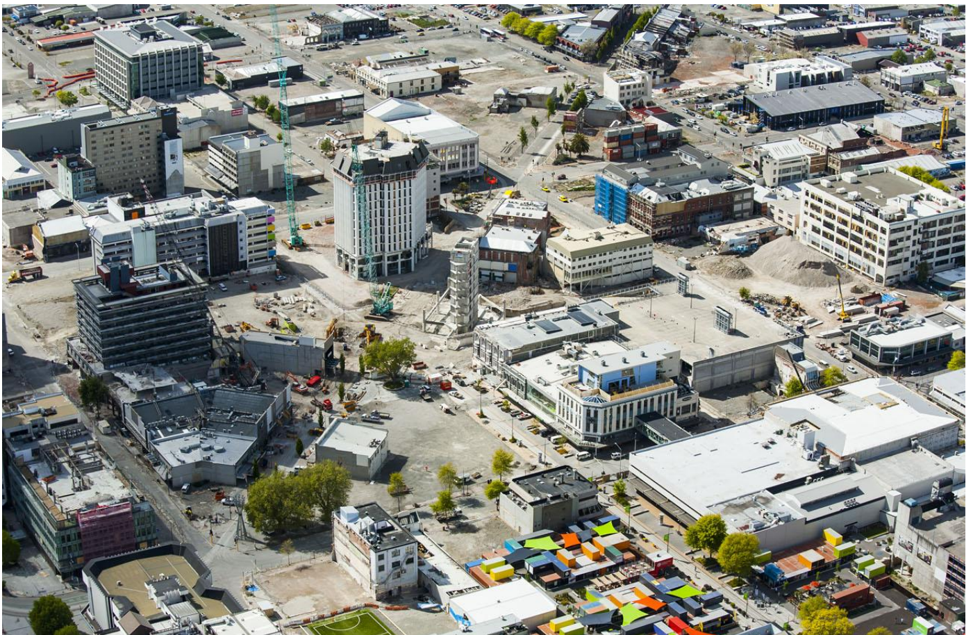
Looking southeast down High Street from above the old CPO with the Restart Mall and Ballantynes lower right. The Westpac building (centre) is in the final stages of demolition. The orphaned line of trees marks the site of the triangle where formerly stood the vibrant shopping area of Poplar Lane. Since September 2012, 1350 buildings in the city centre have been partly or fully demolished including 174 of the 585 of the city's listed heritage buildings.
