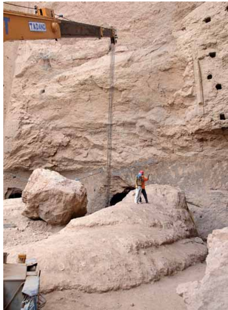
Removal of rock fragments near the uncovered feet of the Western Buddha (photo: B. Praxenthaler)
