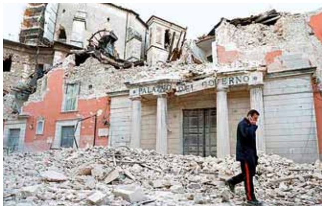
The Palazzo del Governo after the earthquake
