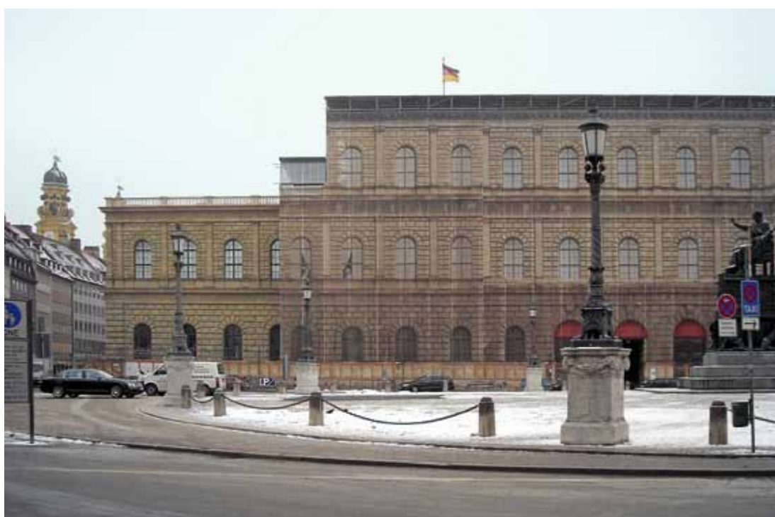
Munich, covering in front of the façade of the Residence (photo: I. Cisek)
