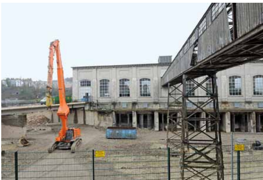
Rheinfelden Power Station (photos: K. Beretta, November 2010)
