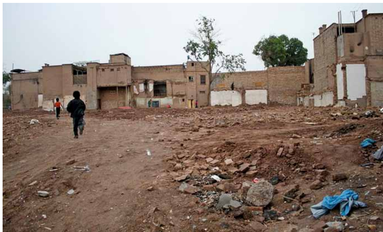
Partially destroyed buildings in the Old City
