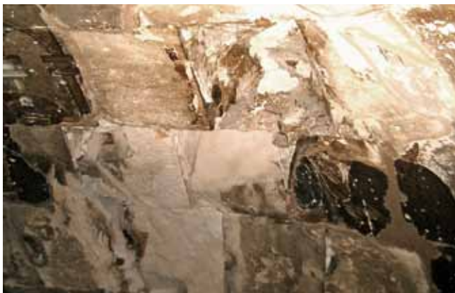
Sioni Church, vault of the south conch with fallen-off cap stone: the mortar shows an imprint of the lost stone trapezoidal in its cross section (photo: Barthel & Maus)
