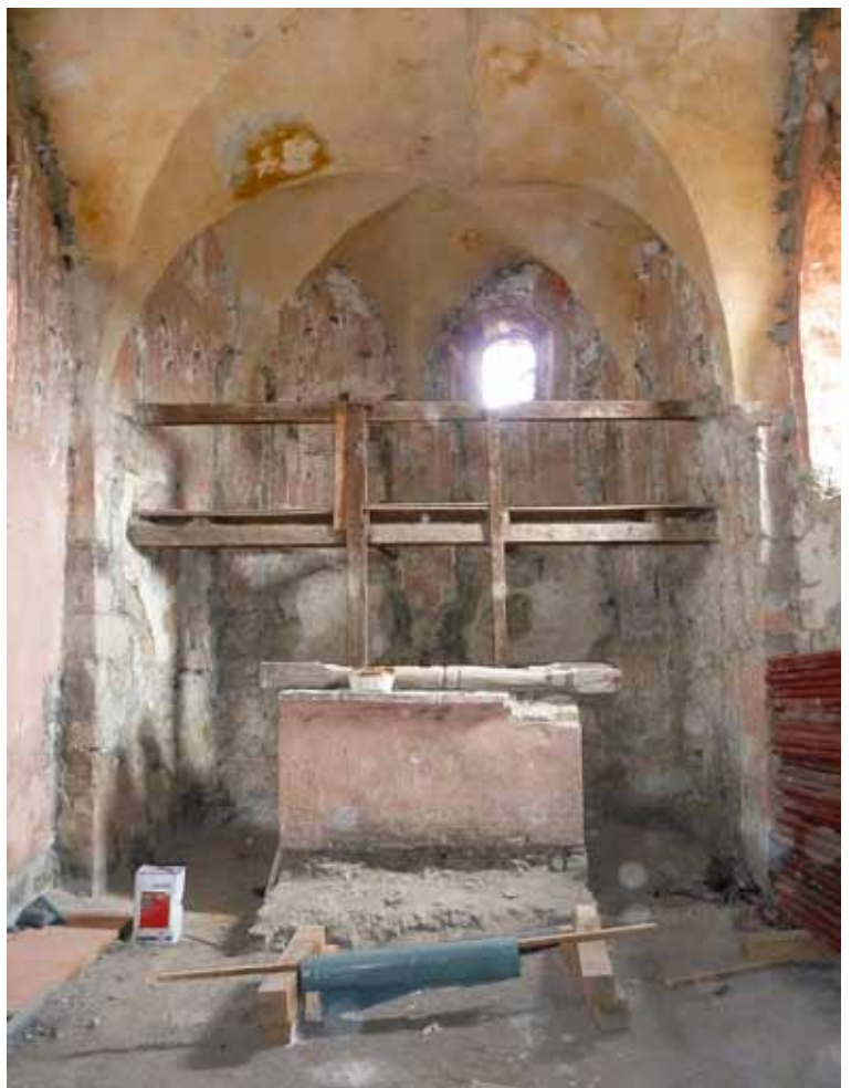
Drăușeni (Draas), church interior in a state of neglect (photo: C. Machat)
