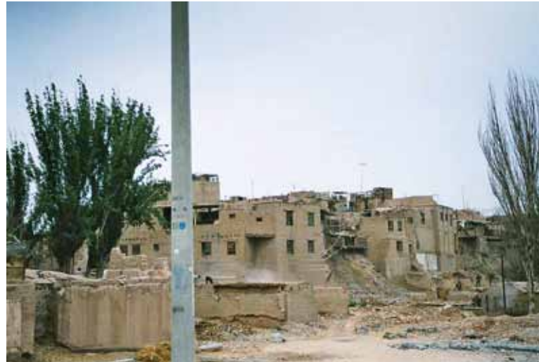
Partially destroyed buildings in the Old City
