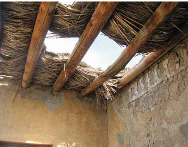
Erebouni Fortress, damaged wall paintings
