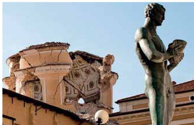
L'Aquila, Santa Maria del Suffragio, the destroyed dome
