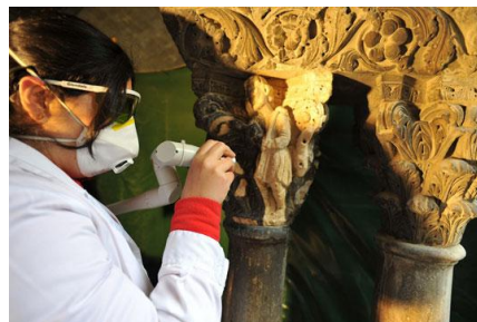
Conservator Vivi Pouli conducting small tests at France's Cloister of St. Trophime with UV and IR laser cleaning device.
