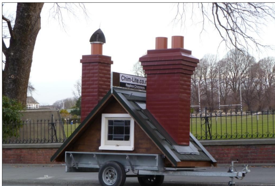
Photo: Emma Reynolds Spotted in Papanui Road, Christchurch, Chim Lite's answer to the toppling stack – a light weight replica in Color-Cote steel described by the manufacturer as "an approved solution by EQR Fletchers [sic] for replacing chimneys in Canterbury."
