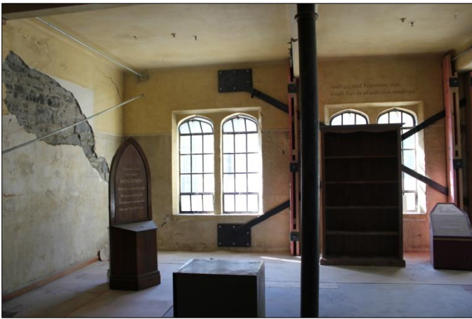
Above & Below: Temporary bracing in the former Belgian Beer Cafe tenancy.
