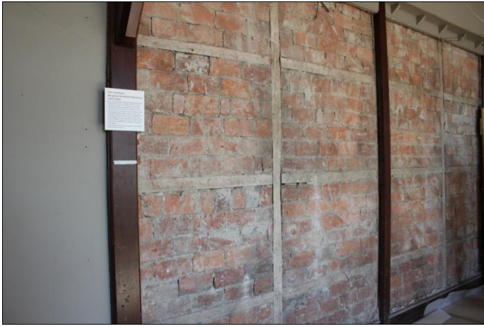
Above: Removal of later wall cladding reveals brick nogging in one of the upstairs office.
