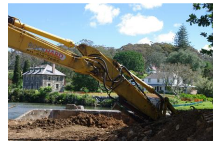
Removing the bridge, Kerikeri Basin
