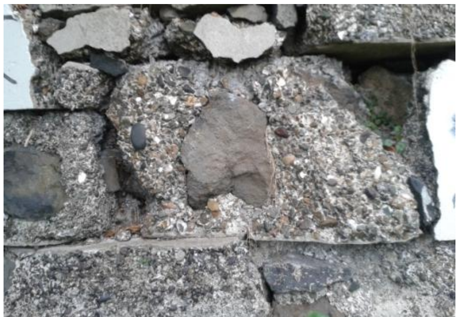
Beach aggregates, shell and 'plums' of basalt feature in the mix used in Logan Bank's walls, now reused as retaining walls for the street above.
