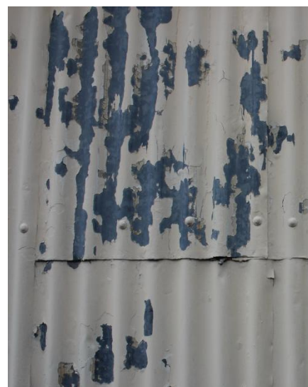
Below: Corrugated iron cladding on the original building
