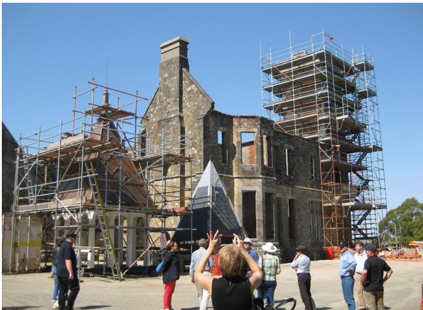
Above right: Burra Burra Railway Station. Below: Marble Hill. (1878) under restoration
