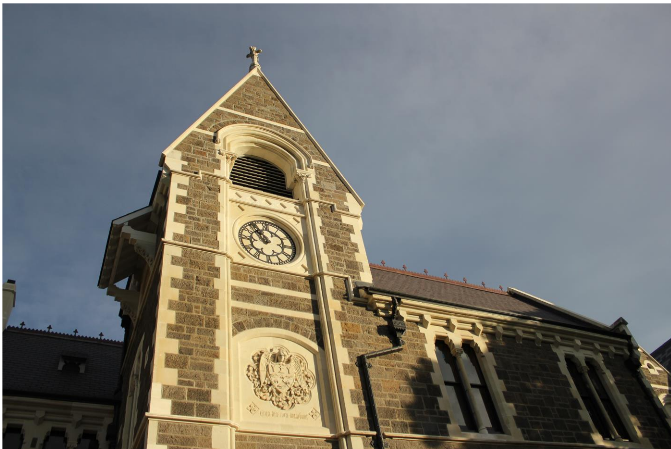
Above: The restored The Clock Tower is Canterbury College's first stone building, designed as a tribute to the Christian Oxbridge tradition. Built of Port Hills basalt and Oamaru limestone, the Clock Tower has a tiled entrance leading on to the north quadrangle and arcades linking buildings. On either side of the Clock Tower, are a number of tiered classrooms which were for English, law, classics, mathematics, modern languages, biology and geology.
