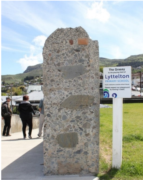
Above left: Concrete with grunt: stone 'plums' and the odd brick revealed in the cyclopean concrete of the old Lyttelton Gaol wall.
