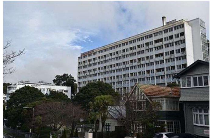
Image Source: McLean Flats and Gordon Wilson Flats, Wellington. Gordon Wilson Flats. Copyright: Heritage New Zealand. Taken By: Blyss Wagstaff. Date: 6/07/2020.
