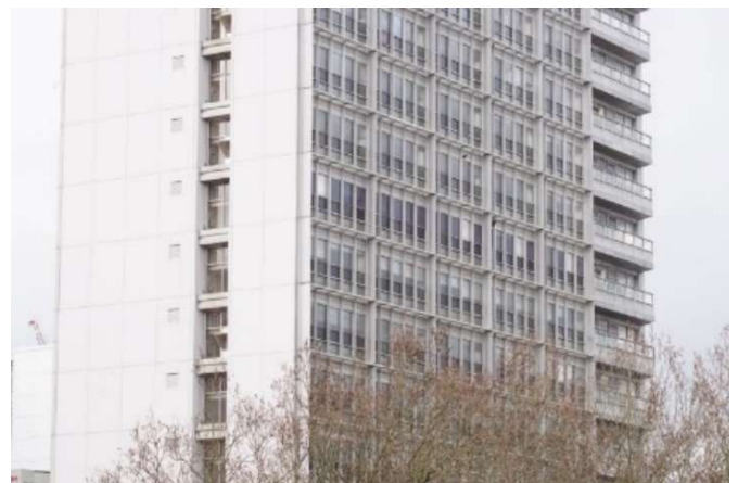
Image Source: Salmond Reed Architects – Civic Administration Building, "Before".
