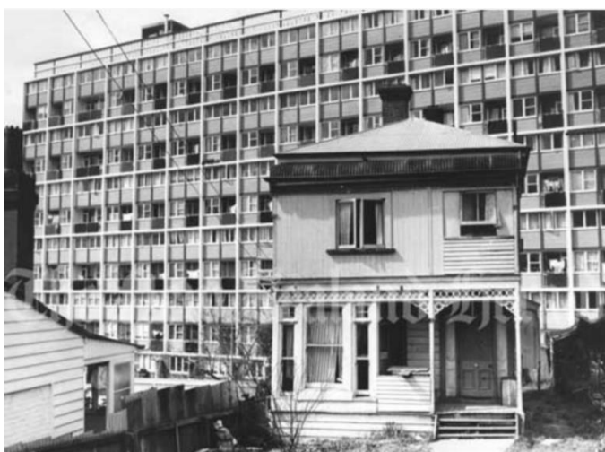
One of the special features of Gordon Wilson flats is the maisonette design (each flat has two floors, one with living and kitchen spaces, and the other with bedrooms). The only other example of this was the Upper Grey's Avenue flats, in Auckland, here deliberately contrasted against the old Victorian housing it has replaced. New Zealand Herald . Reference: 120810NZHFLATS.JPG
